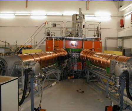
K8 Injector cyclotron 2
